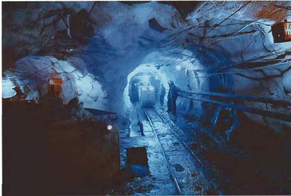
Figure 7. Today, all mining at Mariinsky is done underground. As evident here, the tunnels are quite large, well lit, and well equipped.
