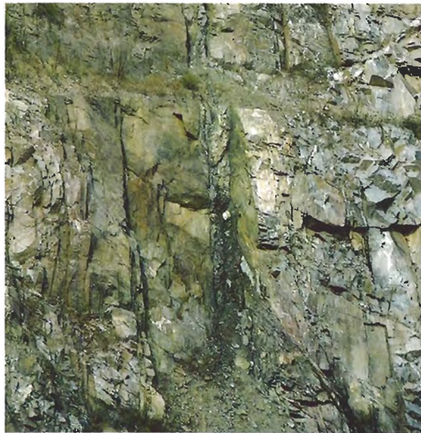
Figure 6. The highly serpentinized Victory No. 2 dike can be seen in the wall of the open-pit mine.
