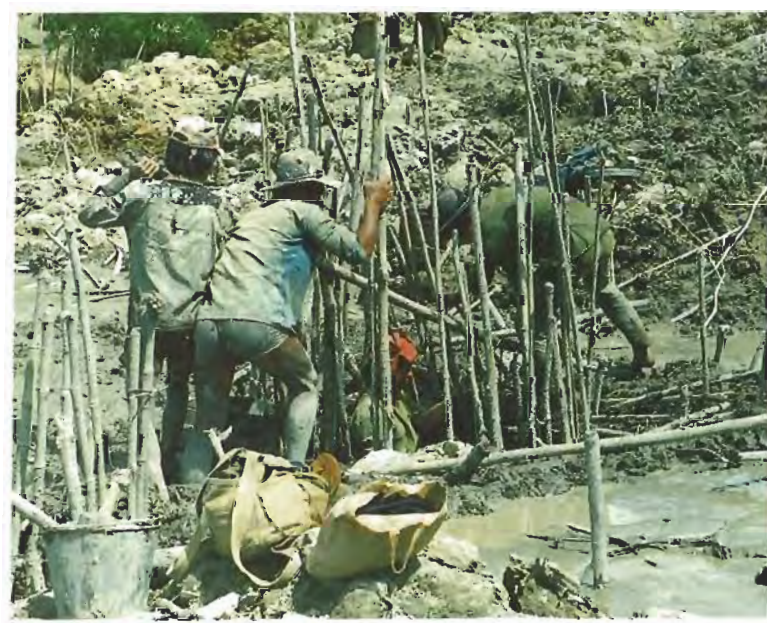
Figure 9. At Quy Chau, pits may be dug as deep as 7 m to reach the gem-bearing gravels, and are reinforced with bamboo poles. Photo by C. Mora.
