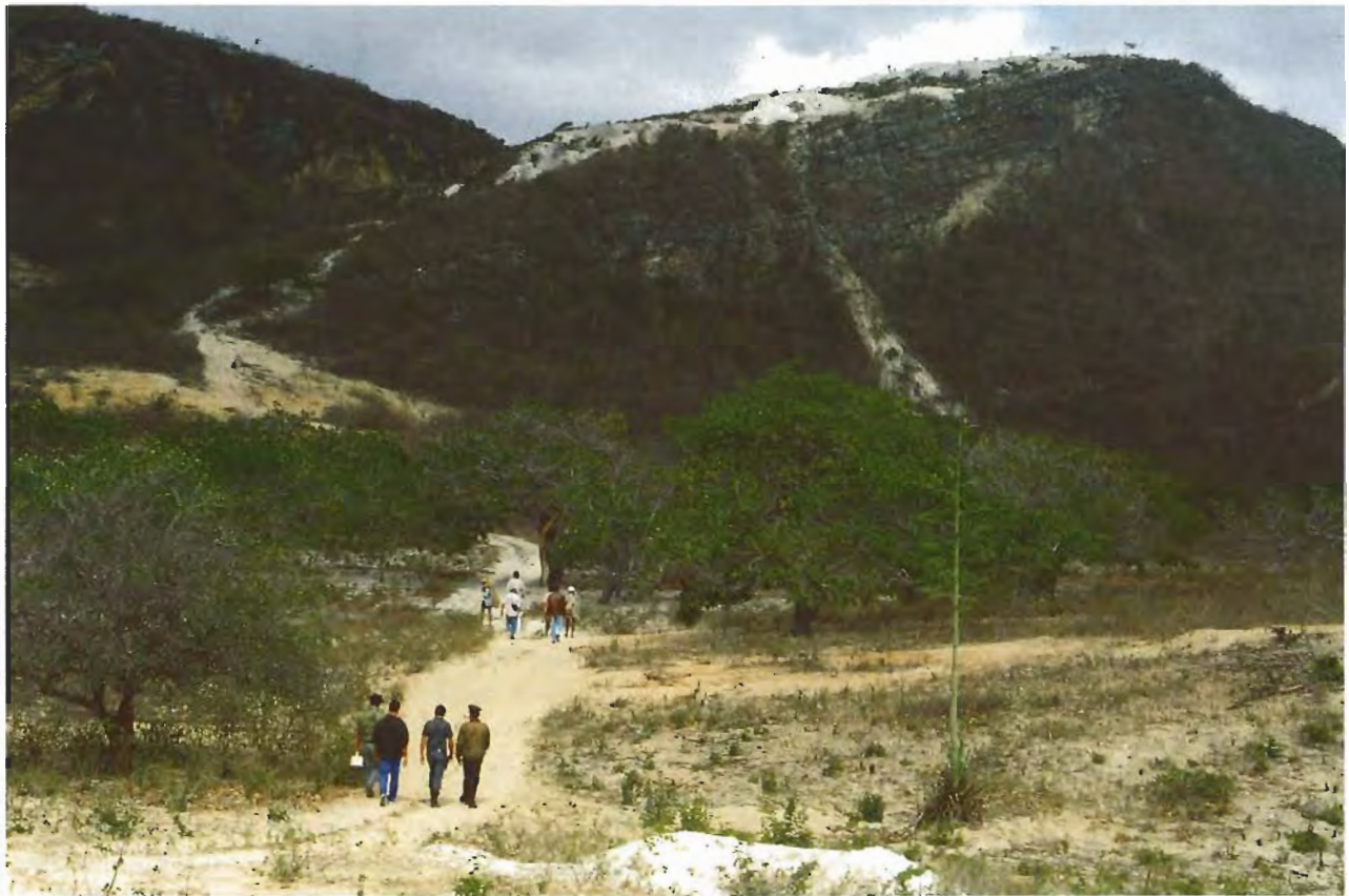
Figure 3. The Mina da Batalha workings can be seen here at the top of Serra da Frade, a hill composed of gently dipping beds of gray quartzite. Dumps of decomposed white rock mark entrances to the mine shafts that have been dug into the weathered pegmatite. Photo, taken August 1990, by Brian Cook.
