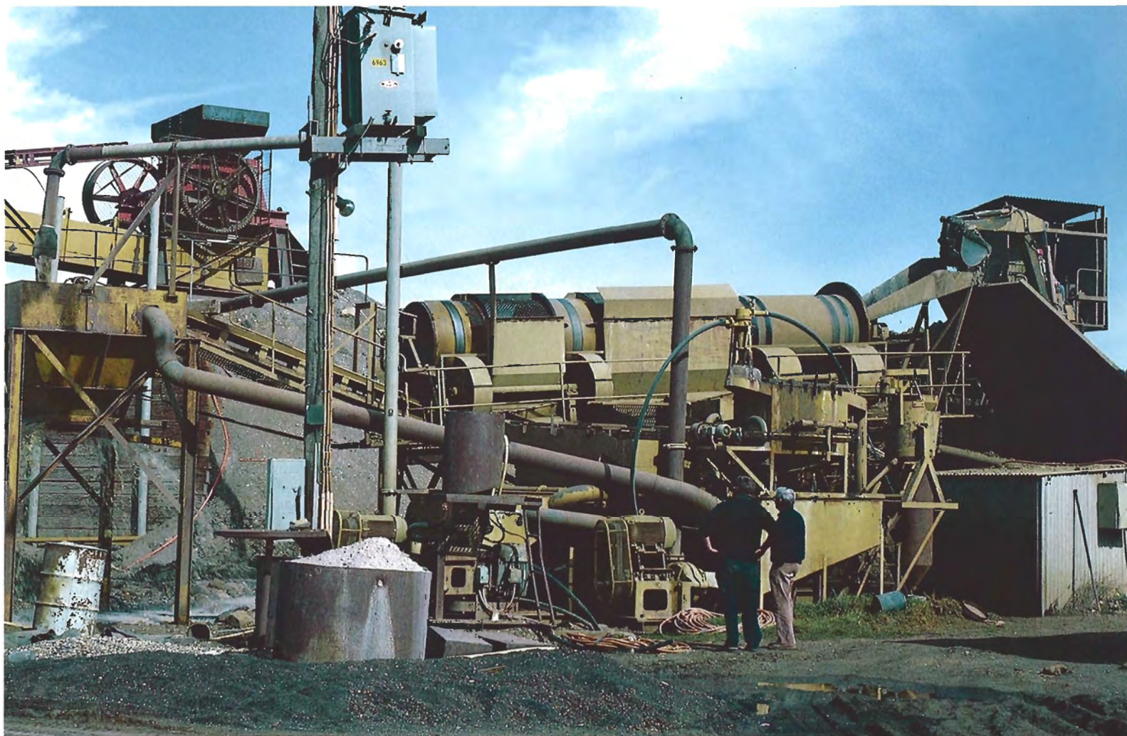
Figure 5. A mechanized processing and recovery plant at Kings Plan, Inverell, in the New England fields.
