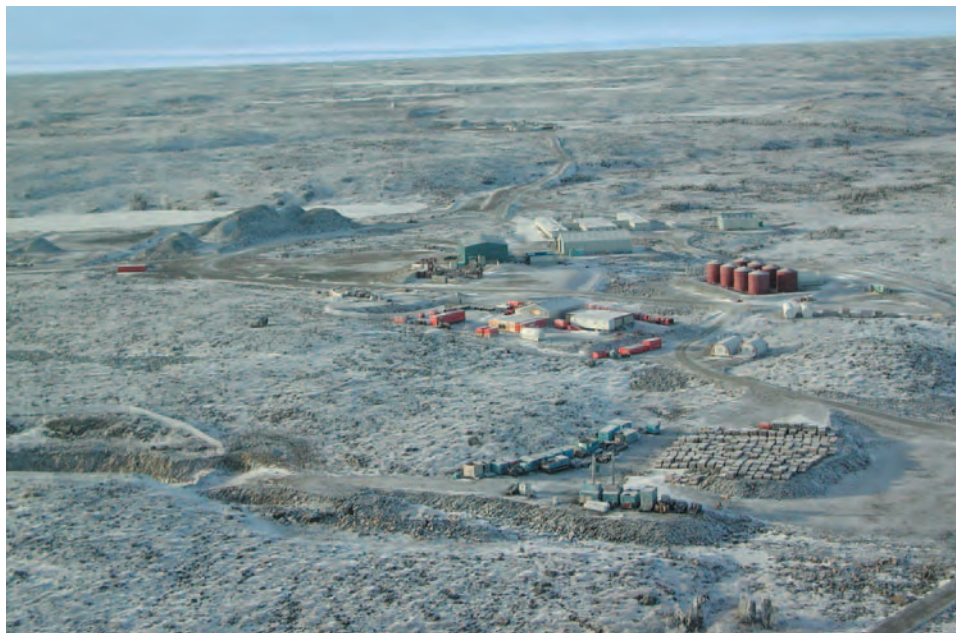
Figure 15. This image of the Snap Lake project, looking southwest, was taken in October 2001. The rock pile on the left rear is an ore stockpile, and the green building is the processing plant. The white buildings house offices and accommodations. The portal to the underground workings is located just to the left foreground of the processing plant, near the elongate orange container. Courtesy of De Beers Canada.
