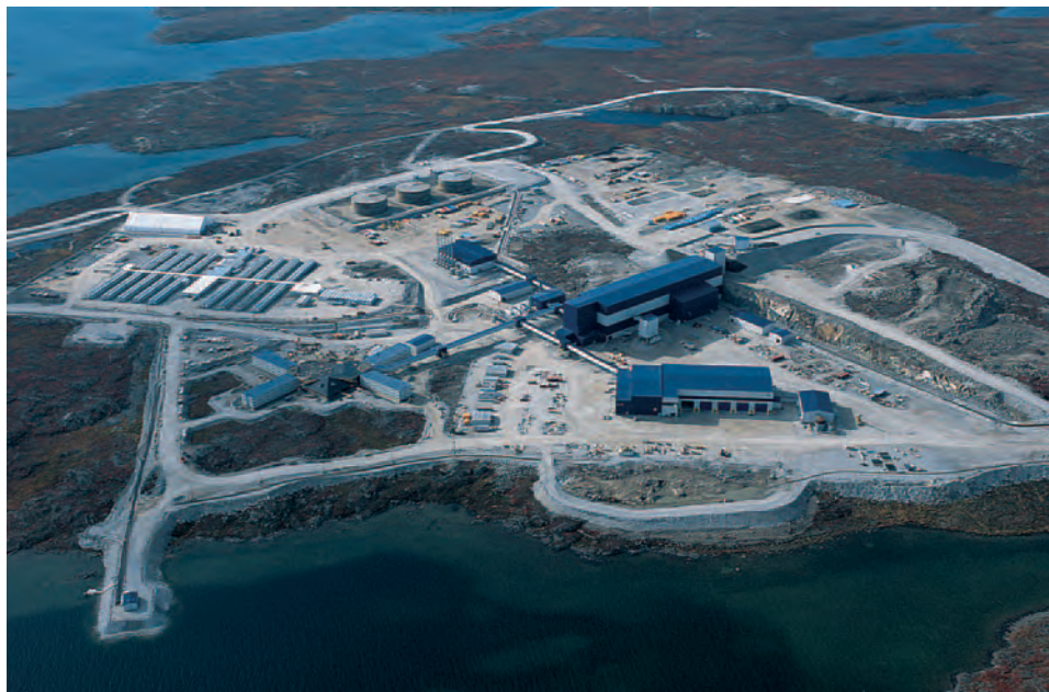
Figure 13. This aerial view of the Diavik mine was taken in September 2002. The large (11 story) building in the center is the processing facility, where diamonds will be separated from the kimberlite host rock. The building to the lower right serves as the maintenance and administration center. In the lower left is the permanent accommodations facility, and above it (with the smoke stacks) is the power plant. Photo by Jiri Hermann; courtesy of Diavik Diamond Mines Inc.
